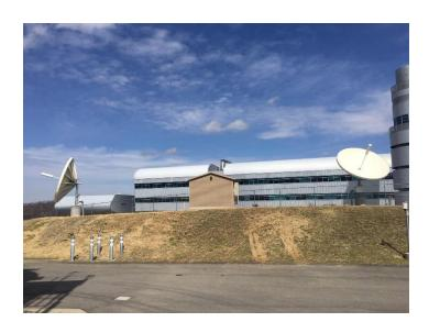
NOAA seeks to replace the omni-directional backup pilot uplink antenna currently installed on the roof of CBU with two 3.8m parabolic antennas similar to the primary pilot uplink antennas at WCDAS.
